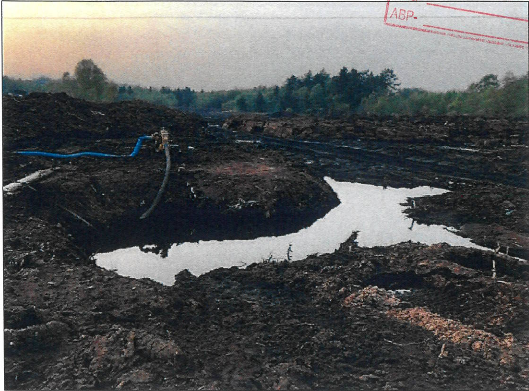
Figure 8: Photograph of pump draining water from the site - discharge licence not in place
